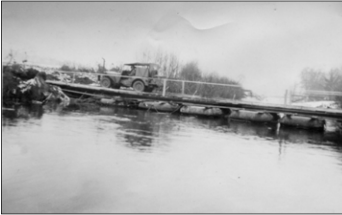
(above) Bridge built on New Year's Day 1945 by B Company (Frank Lembo)
